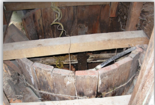
Examples of unused wells: drilled well with corroded casing (above); open dug well (below).
