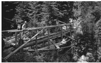
Historical McBey Creek Bridge along Arrowsmith Trail (Photo: BC Archives).
