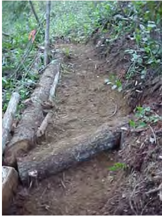
Erosion control measures (Photo: P. Rothermel).
