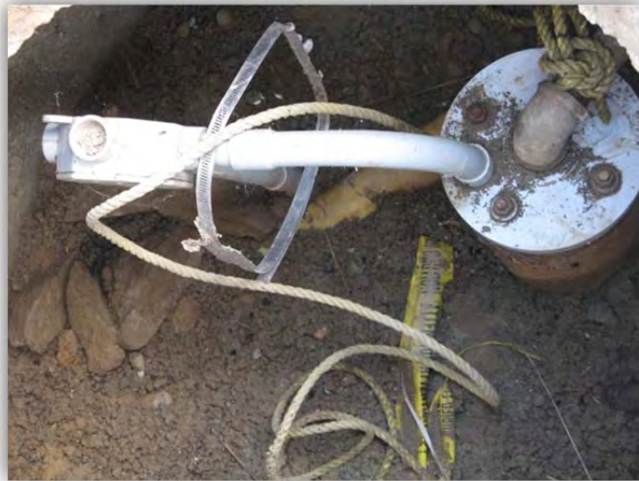
Rollo McClay Wellhead Close-up in 2012
