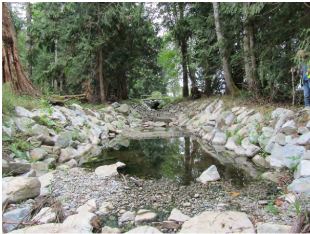
Photo looking east from Bower Road
