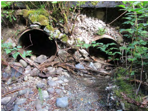
600 mm culverts under Railway
