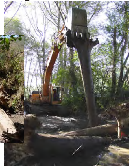
Constructing Log Check Dam
