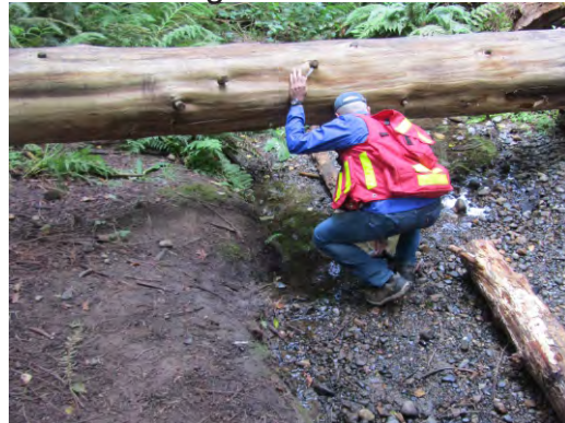
Photo south of Hamilton Avenue
