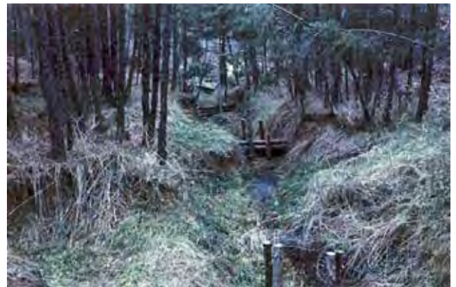
Log Check Dam
