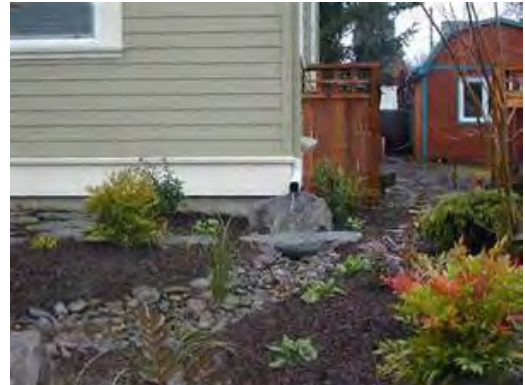
Disconnected Downspout
