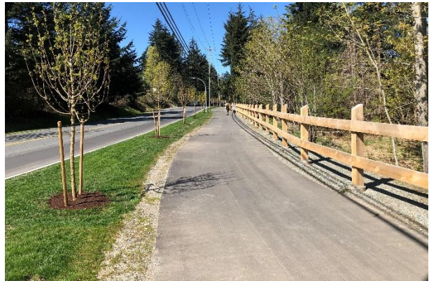
Hammond Bay Frontage Trail Improvements
