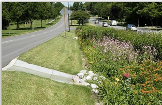
Examples of a rain garden and rainwater harvesting system.
