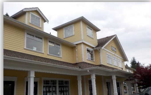
Example of building articulation, varying rooflines & exterior architectural design detail.
