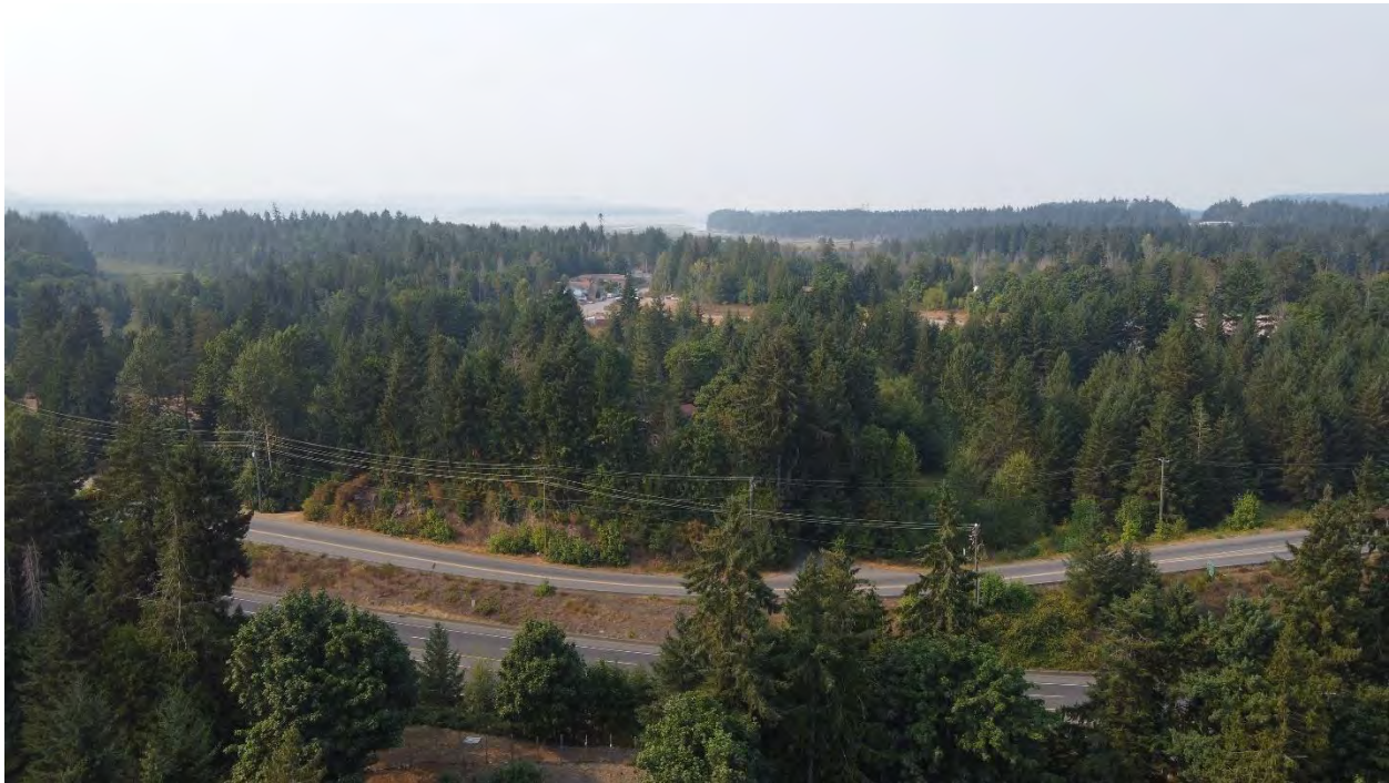
Photo 4. Electrical distribution network near Duke Point Highway.
