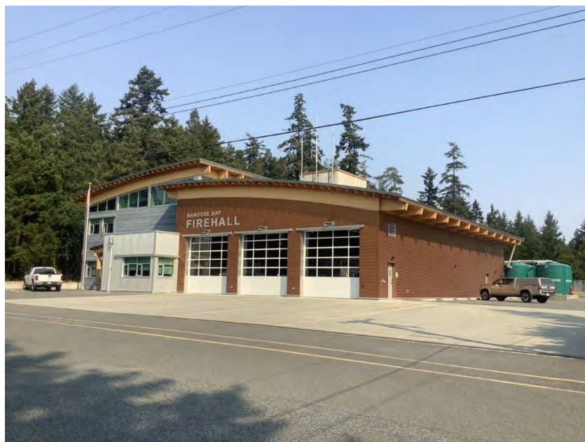
Photo 10. The Nanoose Fire Hall uses FireSmart construction techniques.
