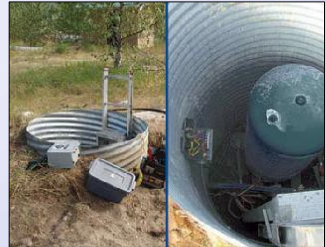
Drilled Wells in Pits
