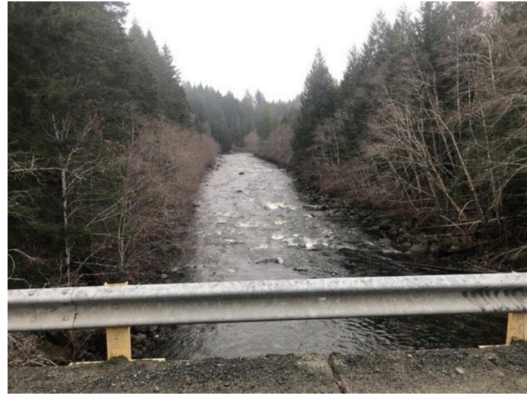
2.) R13 – At Jump Mainline Bridge looking at lower reach
