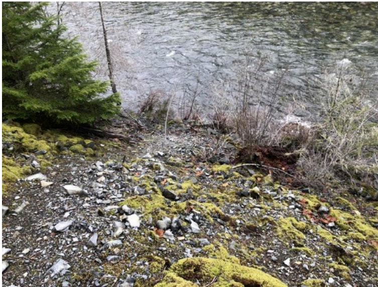
5.) R12- Slide track along rail grade needs planting
