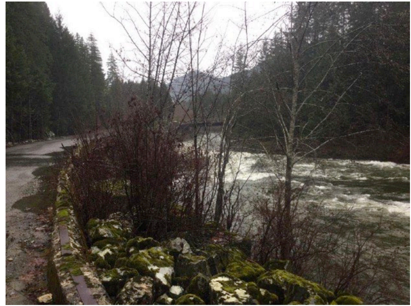
2.) R19 with paved road alongside the confined reach
