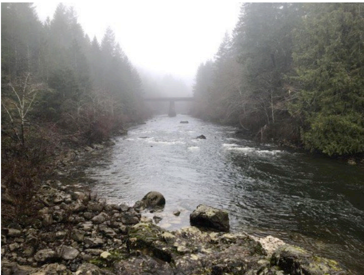
3.) R16 R1 looking up at Bridge with centre span in channel
