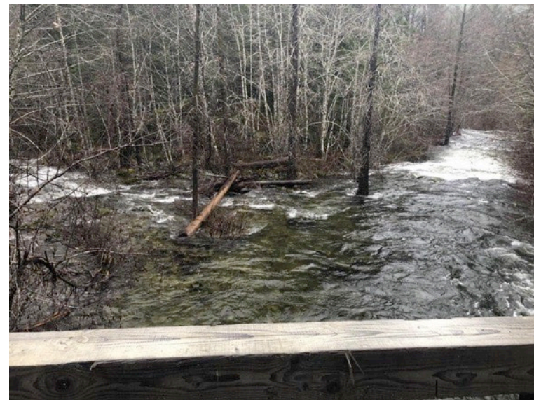
4.) R23 – Sadie Creek at Bridge is flowing through floodplain.
