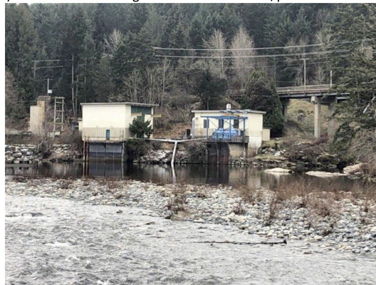
8.) Riffle 8 and Pool 4, pump house at end R4 at Hwy 1.
