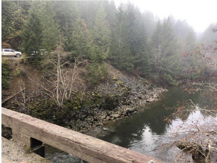
1.) Spawning Gravel placement – possible access site.
