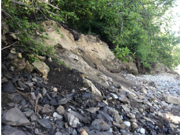
Reach 2 erosion at RDN trail head
