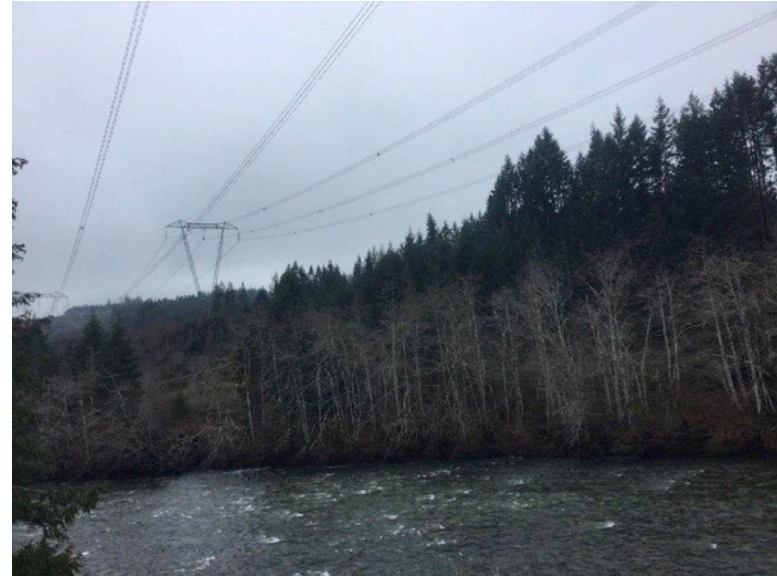
6.) R12- R2 Hydro Line crossing, Riparian is shrubbery/Alder.
