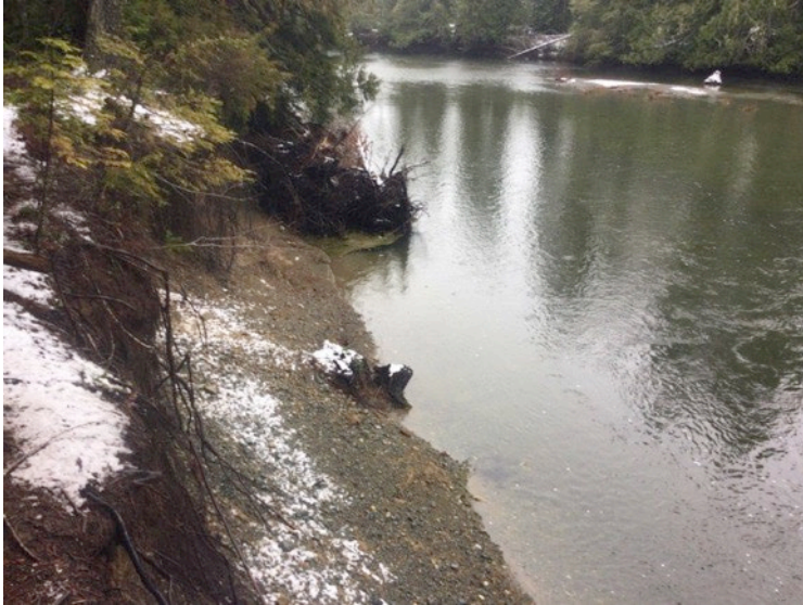
5.) R14-Glide 2 – 20m left bank erosion
