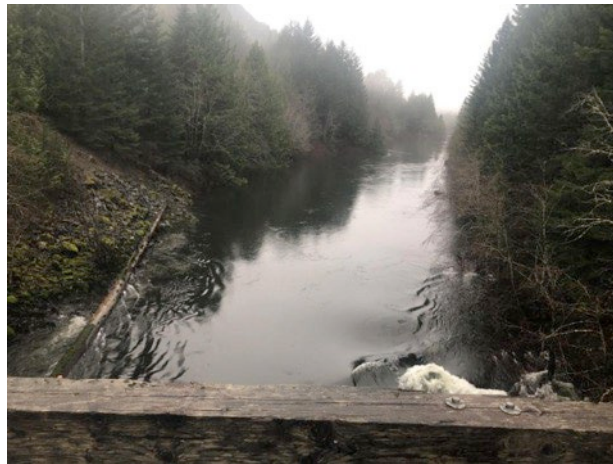
Reach 16 has 80m armoured bank at bridge.
