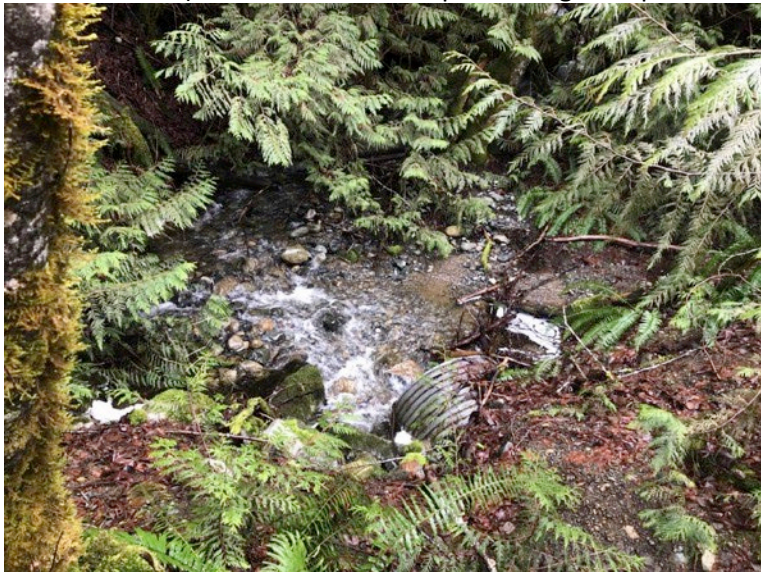
3.) R13 Placemark 9 culvert under rail grade
