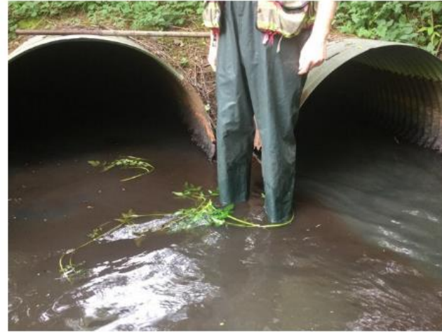
R3 - Rugg Rd Culvert 1
