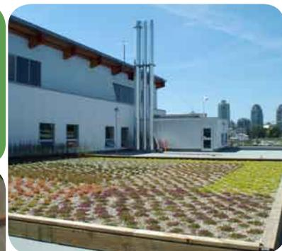
A green roof provides stormwater management and reduces heat island effect
