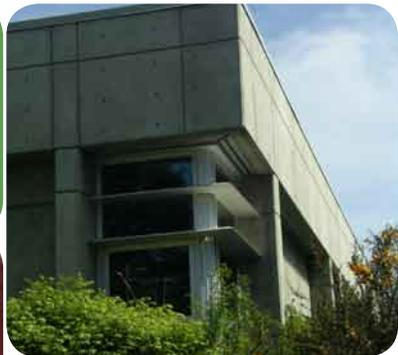
High performance glazing with solar shading
