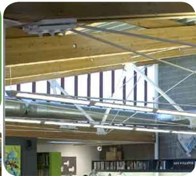
Coating added to clerestory windows filters the sunlight and reduces glare on computer monitors
