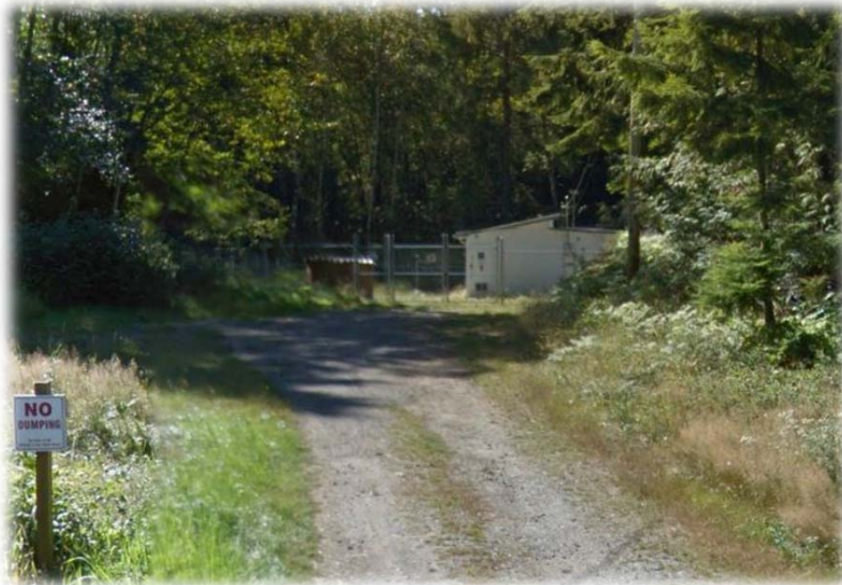
Water Intake Location and Pumphouse
