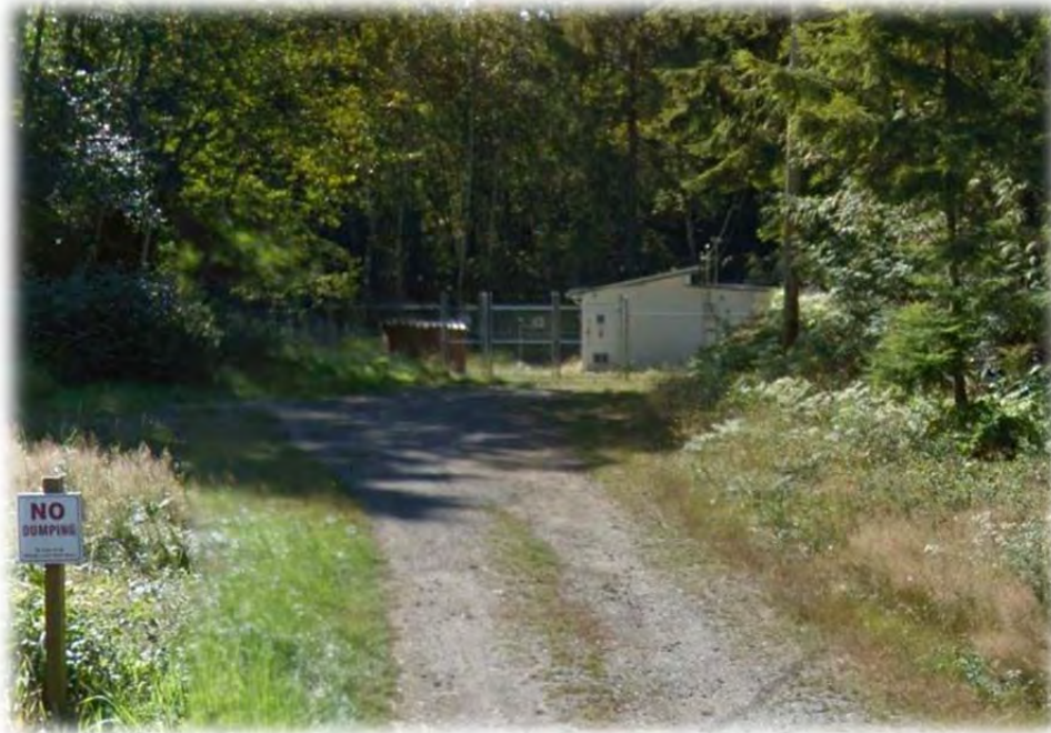
Water Intake Location and Pumphouse
