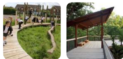
2 BOARDWALK & LOOKOUT focal point for playground, provides sheltered space for sitting, marks edge of playground and forest/wetland
