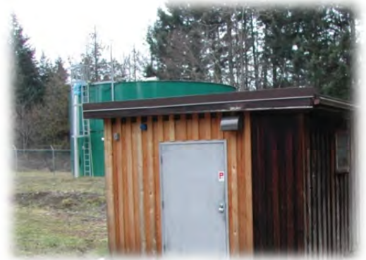
French Creek Main Pump House and Reservoir
