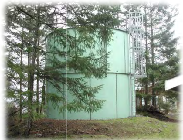
Decourcey Water Storage Reservoir
