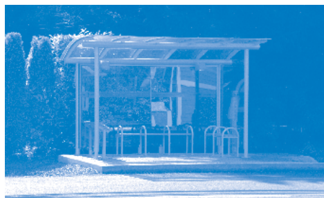
RDN TRANSIT HAS FIVE NEW BUS SHELTERS WHICH INCLUDE LIGHTING AND WHEELCHAIR-ACCESSIBLE PADS.
