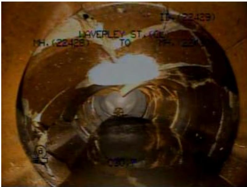
Manhole inspection is another important part of identifying infiltration. Based on similar condition assessment principles to pipes, manhole should be visually inspected to identify cracks and holes that allow infiltration of groundwater, an example of which is shown below.
