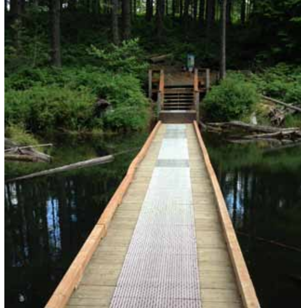
Floating boardwalk at Witchcraft Lake Regional Trail
