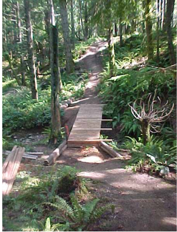
Footbridge under repair
