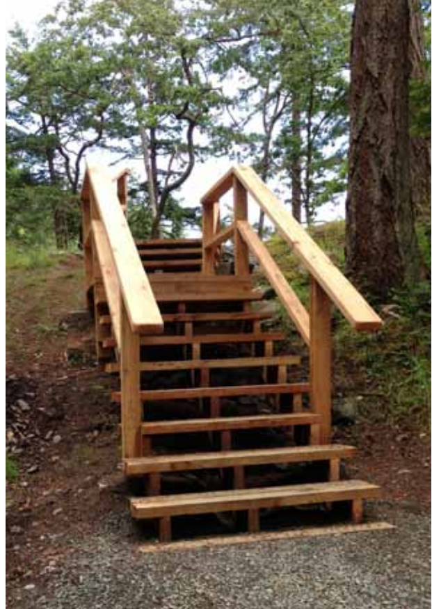
Stairs constructed with stringers from demolition project
