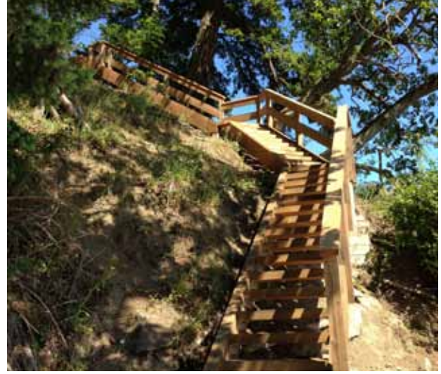
Engineered stairs to beach area
