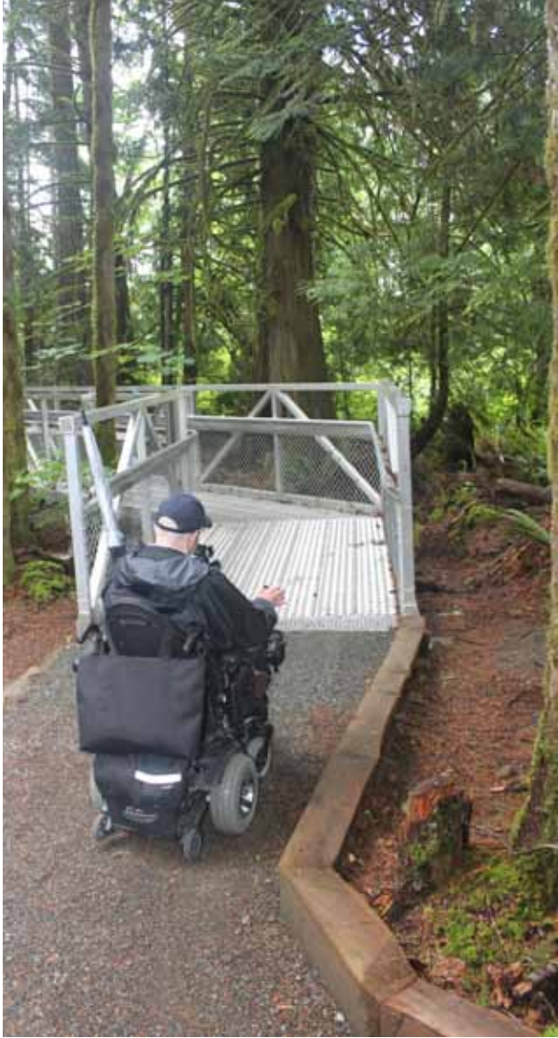
Ledges or lips should be no higher than 15mm (.5 in)
