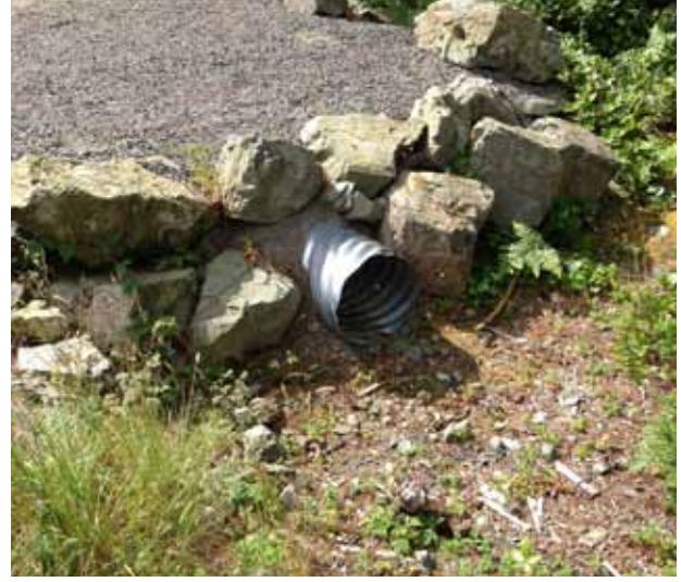
Culvert under parking area
