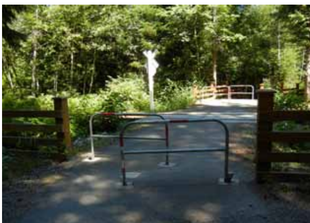
Accessible railroad baffles
