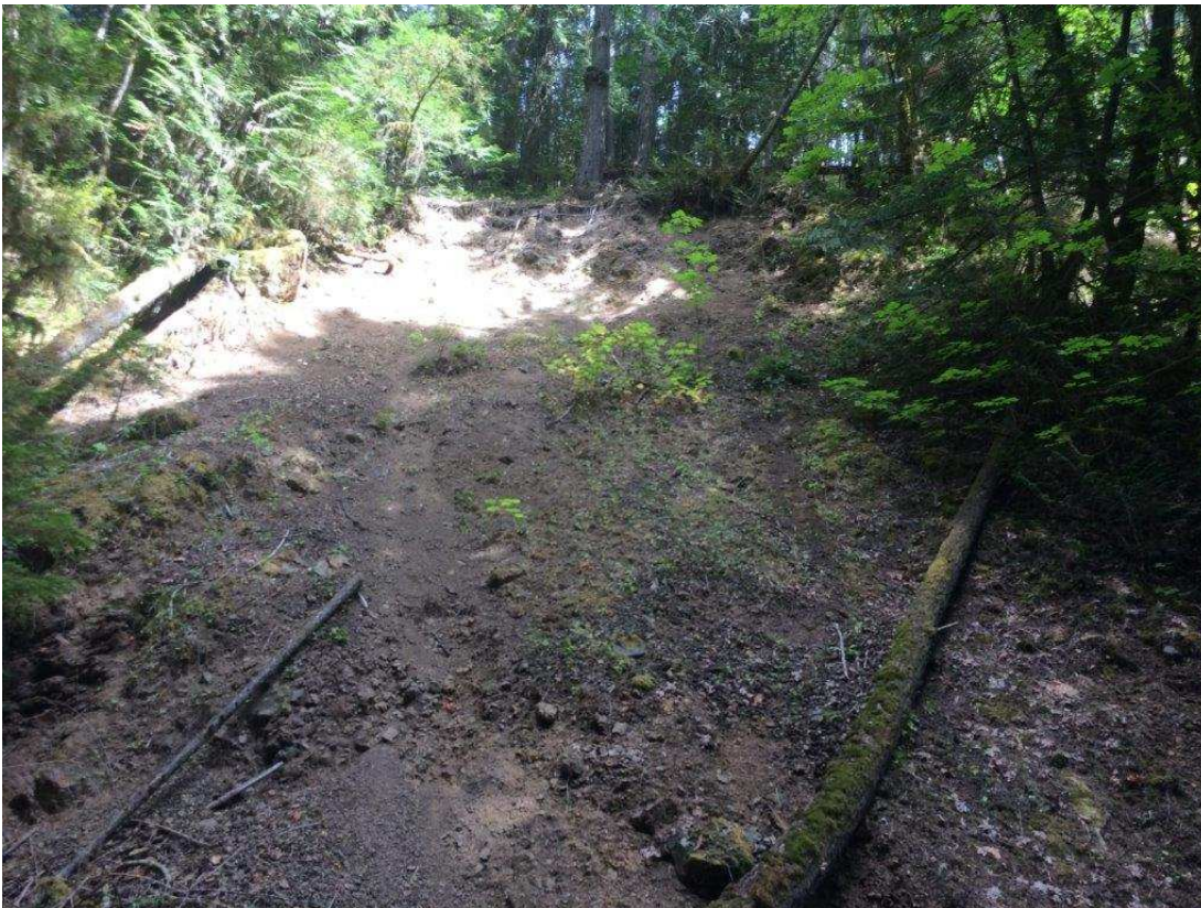
Photo 2: Shallow surficial debris flow failure downstream of log crossing area.
