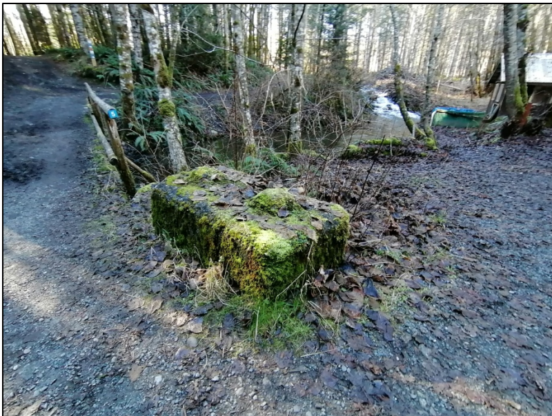
Photo 6: Lock blocks to be removed.
