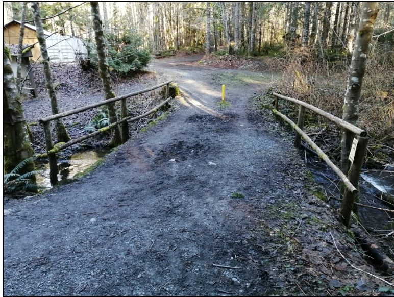
Photo 1: Facing north across the first bridge by the hatchery.
