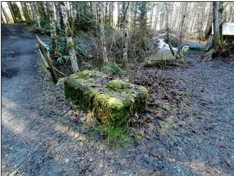
Photo 6: Lock blocks to be removed.
