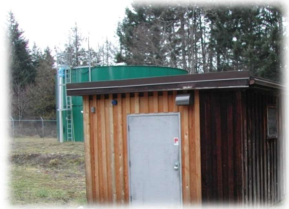
French Creek Main Pump House and Reservoir
