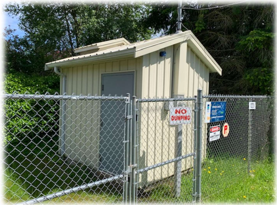
French Creek No.2 Pump House
