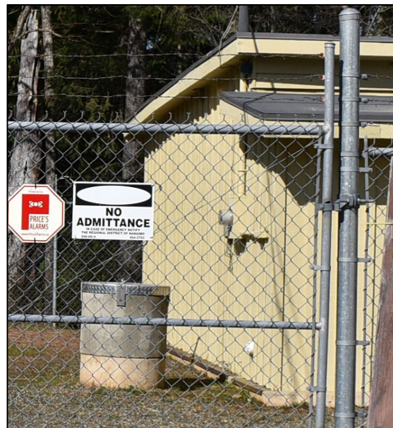
Melrose Well and Pumphouse
