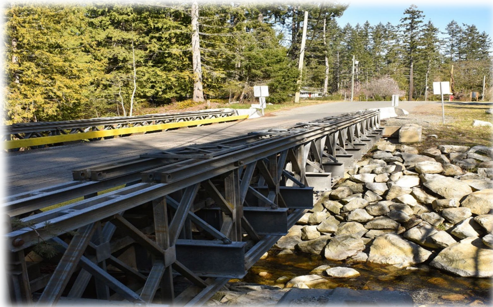
Melrose Road Bridge
