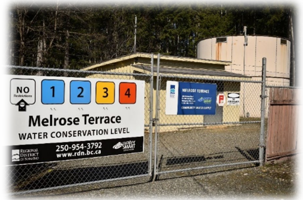
Melrose Pumphouse and Reservoir
