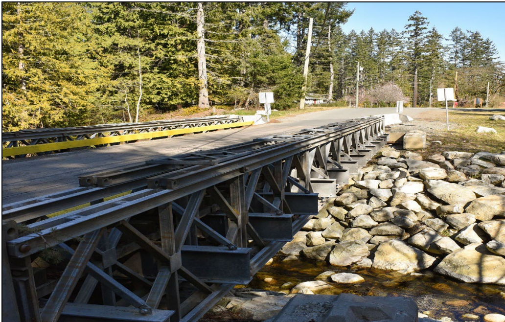
Melrose Road Bridge
