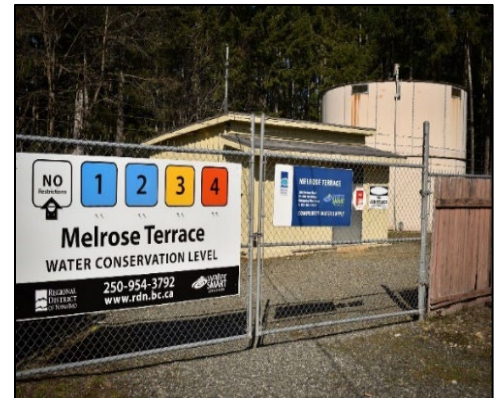
Melrose Pumphouse and Reservoir
