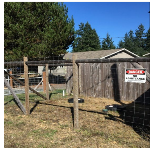
Westurne Heights well site and fence
