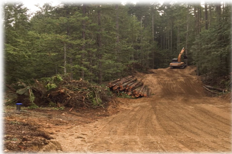
Land clearing and road construction in Whiskey Creek
